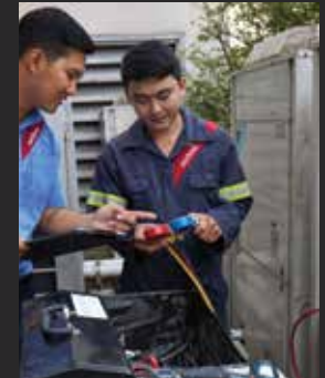
INTEGRATED & TECHNICAL FACILITIES SERVICES
