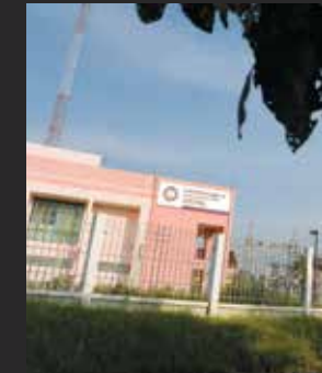
POWER SUB STATION
