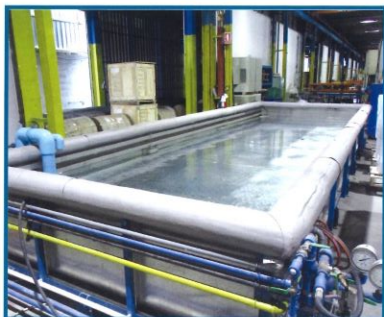
Leak Test Coil 7.2 M.
